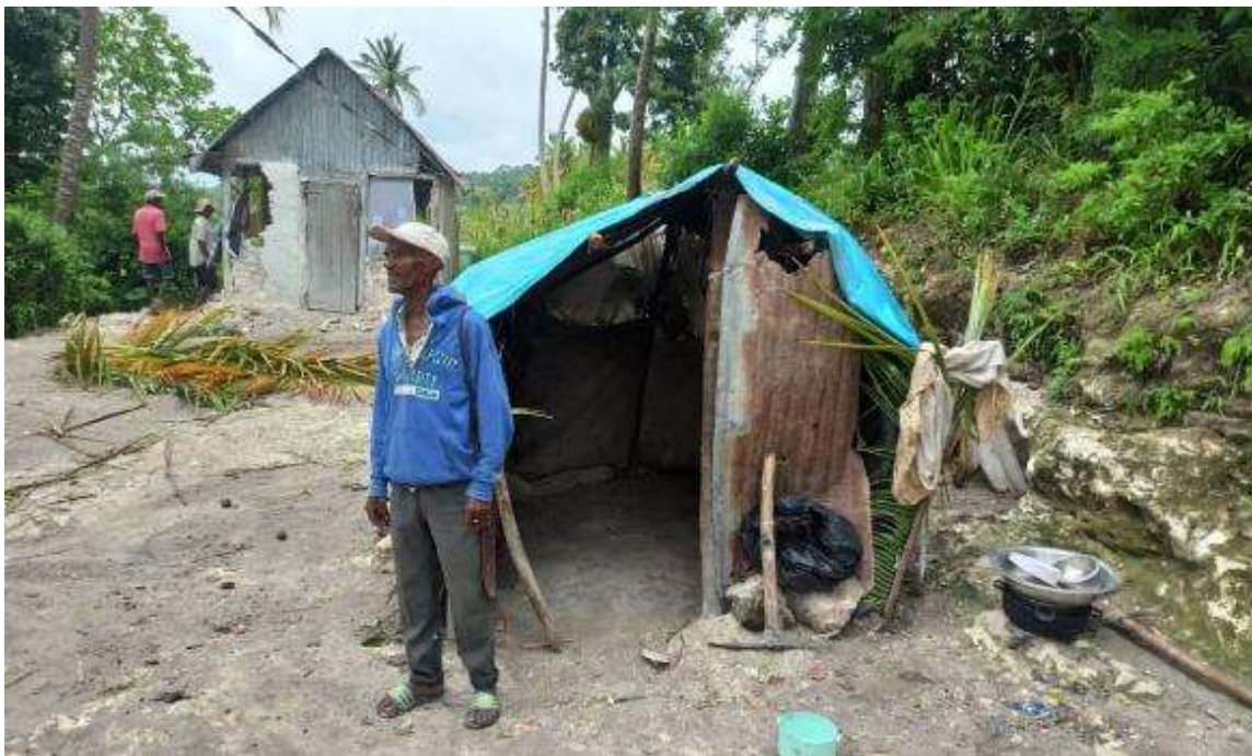
Plastic tarpaulins as a quick roof for the emergency dwellings.
